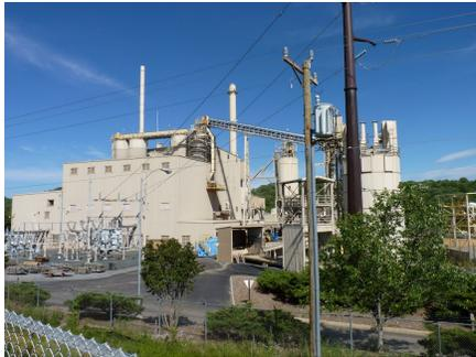
Microfusion has improved the steam header stability and improved the boiler MW control by improved and simplified the overly involved original combustion logics for a recently converted biomass 63MW power generation unit. The improvements include air curve and O<sub>2</sub> changes, air to fuel cross limit changes, Overfire and under-grate air curves recalibration, and the proper fuel master to boiler master integration.
